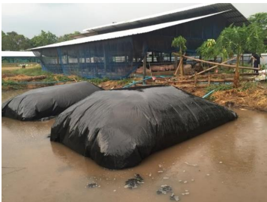
Fig. 1 Elastic balloon containing raw biogas
